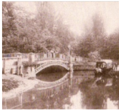
The Hack - Bridge c.1895
